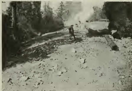
Fire Trail Built in Humboldt County Redwood Park
